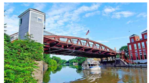
Erie Canal Lift Bridge
