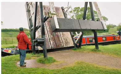
Llangollen Lift Bridge
